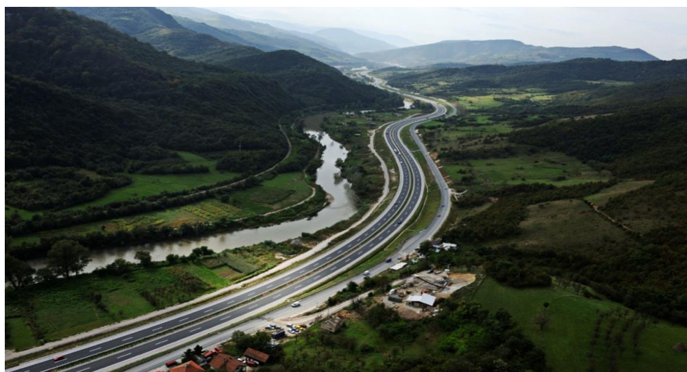
Newly built motorway on the Tarčin – Sarajevo – Zenica section on the Mediterranean Corridor (Vc) in Bosnia and Herzegovina.
