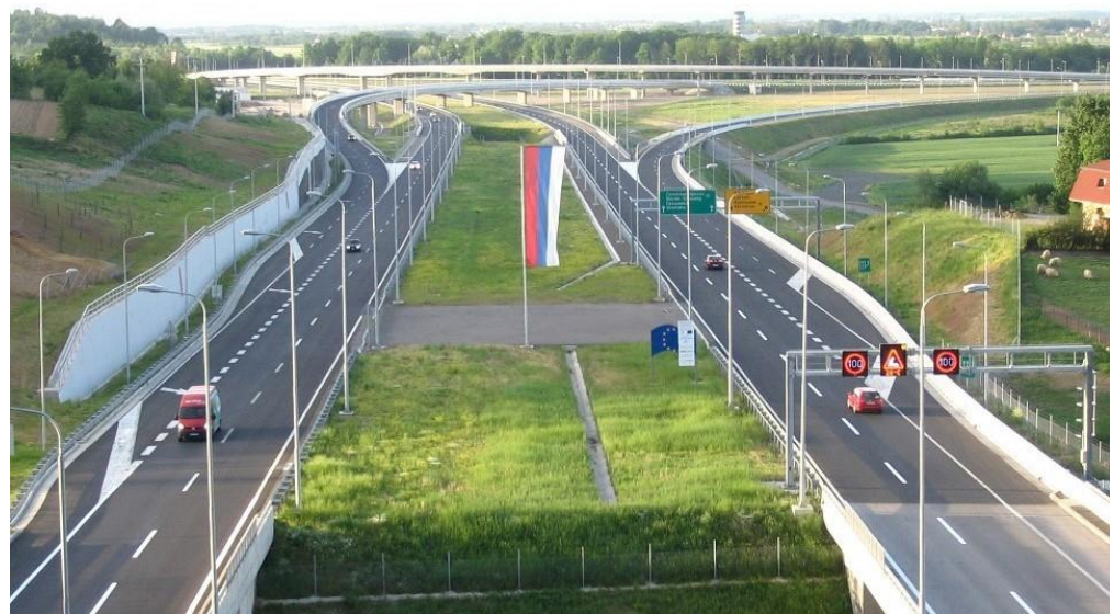
Newly built Mahovljani Interchange on the Banja Luka – Doboј motorway in Bosnia and Herzegovina. (c) JP Autoputevi Republike Srpske.
